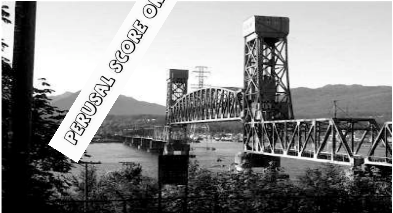
Second Narrows Bridge 1957
